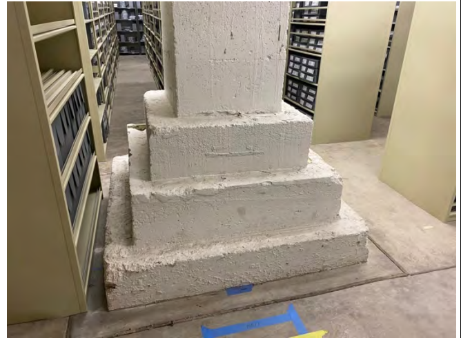
PHOTO 2: Asbestos Containing Concrete Wall/Column Coating
