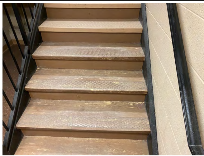
PHOTO 12: Asbestos Containing Stair Tread Adhesive
