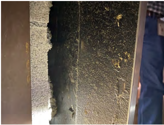
PHOTO 3: Asbestos Containing Elevator Frame Coating
