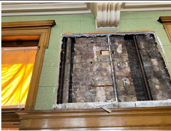
PHOTO 15: Asbestos Containing TSI-Aircell Lagging
