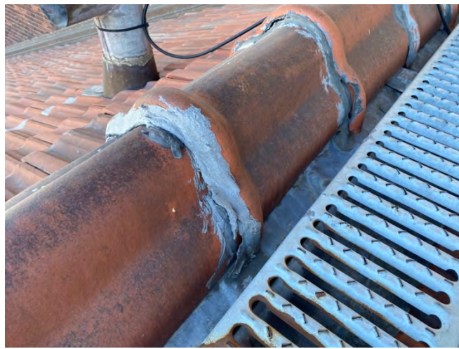
PHOTO 8: Asbestos Containing Black Roofing Sealant
