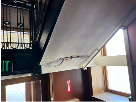
PHOTO 45: PLASTER UNDER STAIRS
