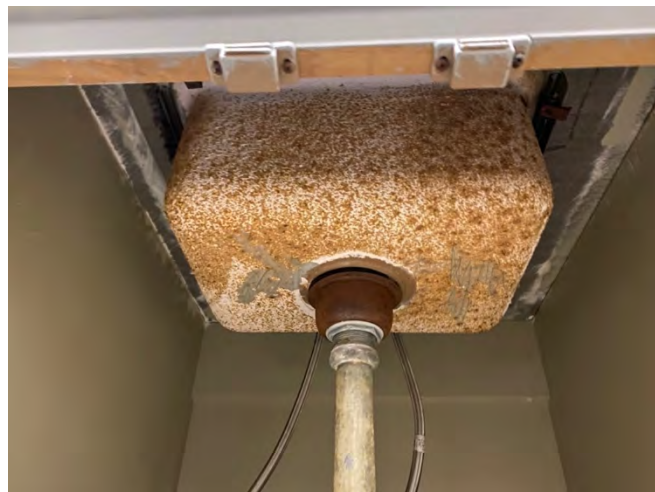
PHOTO 10: Asbestos Containing White Sink Undercoat
