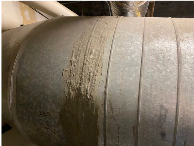
PHOTO 13: Asbestos Containing Green Duct Sealant
