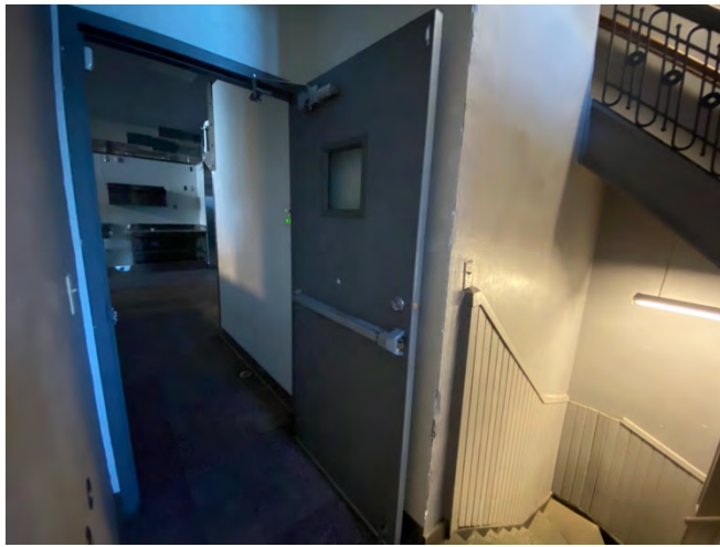
PHOTO 19: Assumed Asbestos Containing Fire Rated Doors
