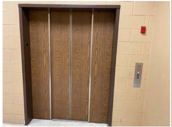
PHOTO 4: Asbestos Containing Elevator Frame Coating
