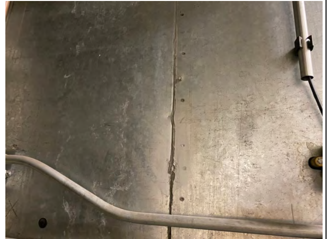
PHOTO 14: Asbestos Containing Gray Duct Sealant
