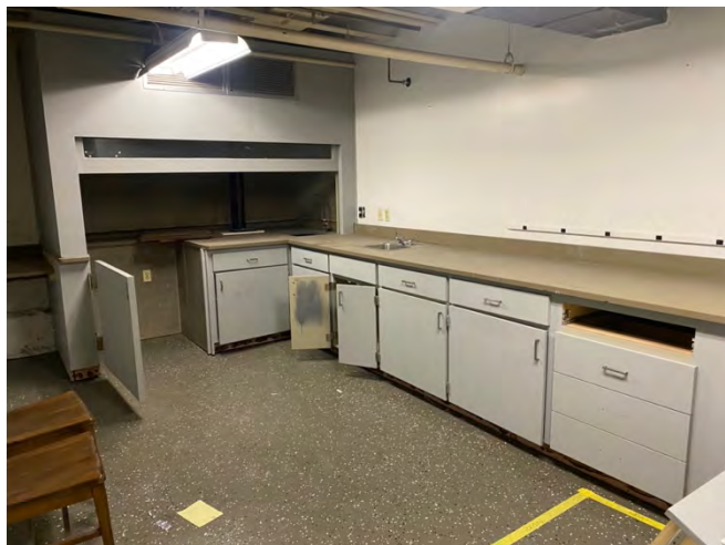
PHOTO 9: Asbestos Containing Fiber Cement Fume Hood & Counter Top
