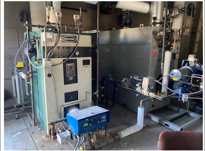
PHOTO 20: Assumed Asbestos Containing Boilers
