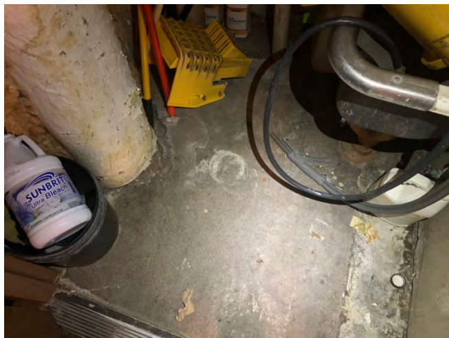
PHOTO 5: Asbestos Containing Sheet Vinyl & Mastic
