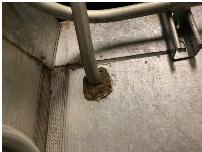
PHOTO 6: Asbestos Containing Brown Putty Wall Packing
