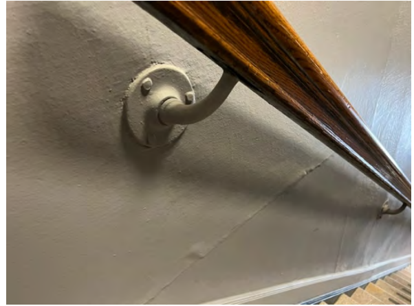
PHOTO 38: STAIR RAIL COMPONENTS
