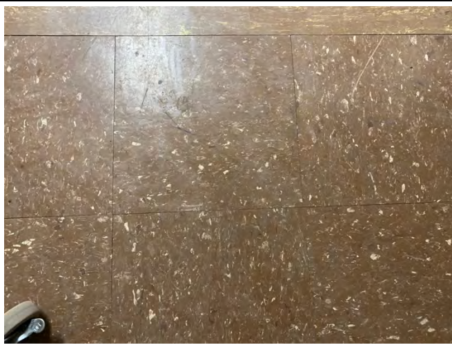
PHOTO 11: Asbestos Containing 12" Vinyl Floor Tile & Mastic
