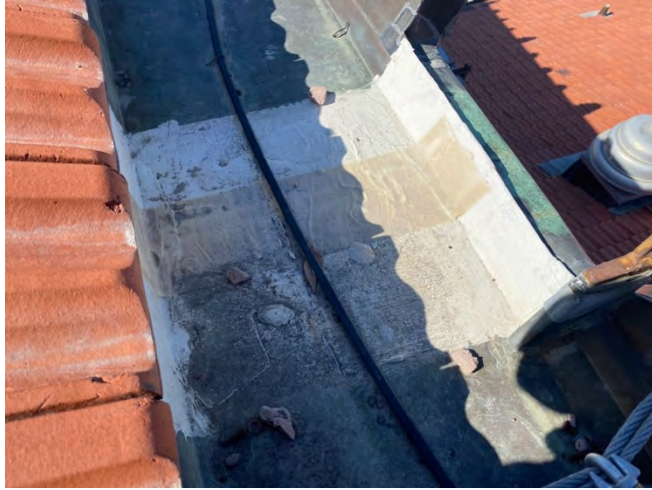
PHOTO 17: Assumed Asbestos Containing Other Roofing Materials (Other Caulks & Sealants)
