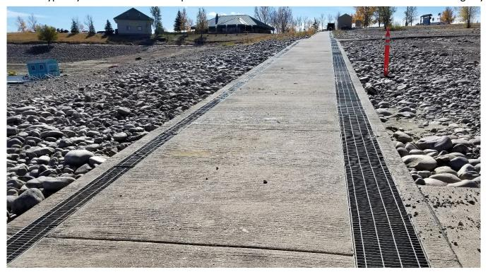
Utility channel pictured above on LEFT side of ramp typically carries sewer utilities for connection to uphill side of Gangway – Gangway should have adjustable legs and transition plate to adapt to varying slope angles
