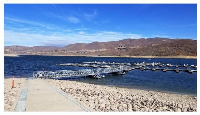
1,000' long sloping shoreline, exposed at LOW water levels, requires long, articulating Gangway capable of being re-located along ramp as docks are moved with changes in water level – Utility channel pictured on RIGHT side typically carries electrical and potable water utilities for connection to downhill side of Gangway
