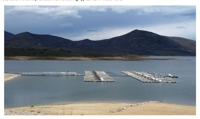
Previous marina gangway was 120 feet long, engineered in (3) sections with 5<sup>th</sup> wheel type connections – Gangway landing relocates along concrete ramp with utility channels as docks are relocated to accommodate changes in water level
