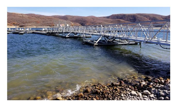
Photo below pictures previous marina T-Head dock with full-service vessel pump-out and waste dump system Note low-level lighting along dock walkway and T-Head dock, also illustrated on attached Drawing – Fuel services may be added to this dock is future
