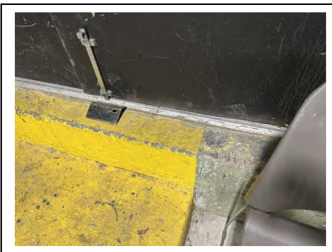
PHOTO 4: Yellow painted concrete contains lead
