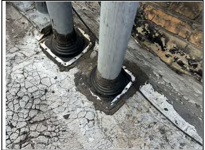
PHOTO 2: Asbestos Containing Roofing Materials
